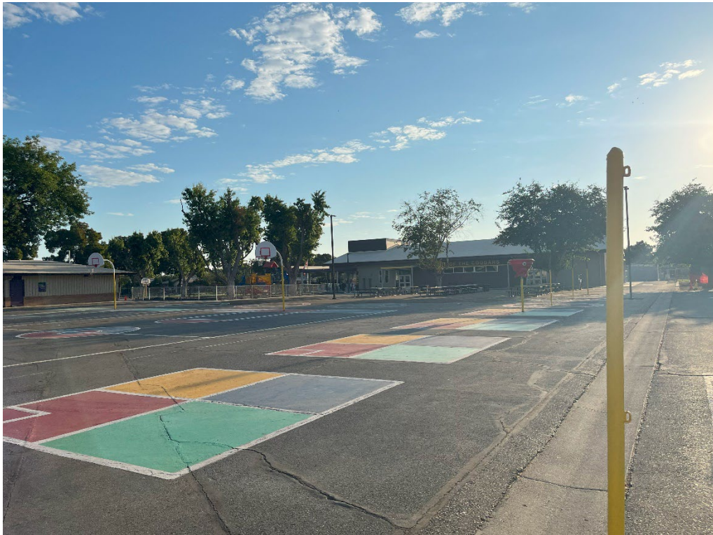
Photo No. 2 – Current site conditions at existing school courtyard, facing northeast.
